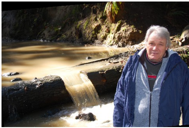
Bob Bridgeman at one of the stormwater and spawning bed installations. Water is diverted away from creek banks, stopping erosion. Gravel is placed behind the dam for Salmon spawning. Thanks for the help from Saanich Parks.
