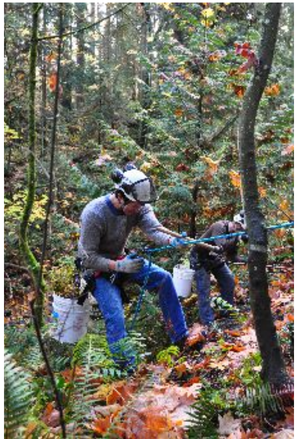
Saanich Parks arborists Dan Fong and Jason Clarke rappel down Douglas Creek bank to help stabilize the cliff with native plants.
