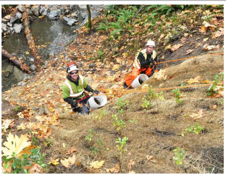
Saanich crews used ropes to plant the steeper creek slopes.
